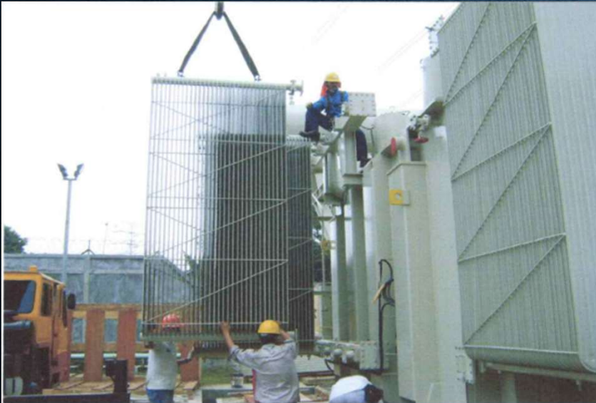
Cooling Radiator installation
