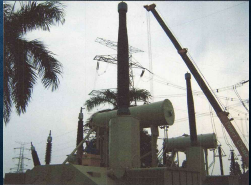
Bushing installation
